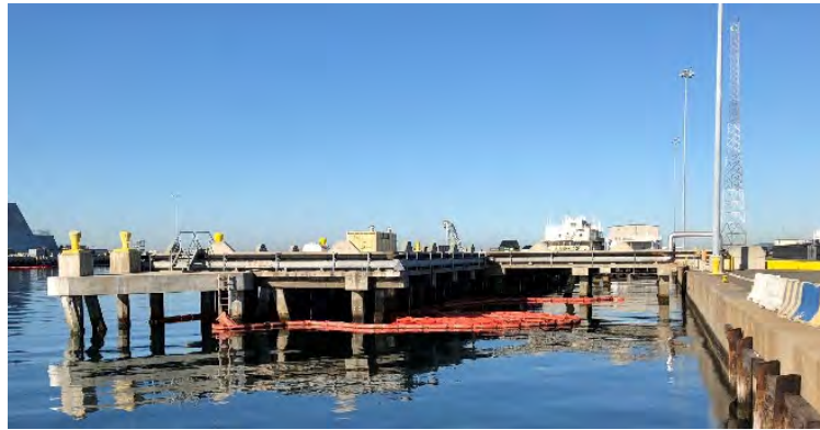
Photo 1. Approximately 2,795 square feet of existing pier deck would be demolished at the south berth of the Mole Pier to facilitate construction of a forward dolphin. The pile-supported extension at the west wharf would also be removed.
