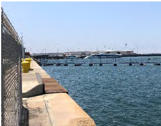
Photo 3. The former Pier 14 was demolished in 2008. This location (shown above) is currently open water with no in-water structures remaining.
